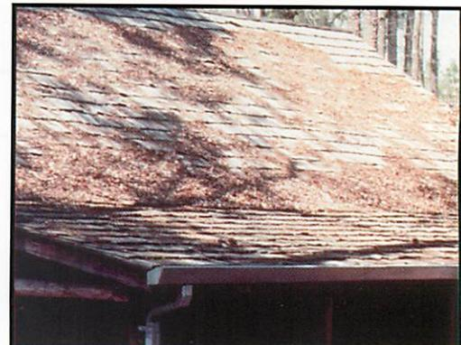
*One spark on this roof could be a disaster. Wooden shingles and leaf litter is hazardous combination.*
